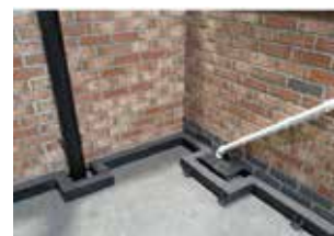
Intrusions for pipework
